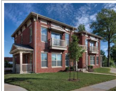
Lexington Housing Authority used New Urbanism design principles in a total remake of 80 acres just east of downtown Lexington that now has nearly 450 new multi- and single-family residences. The five-year project totals almost $100 million. This multi-family structure is in the Grand Oaks section.
