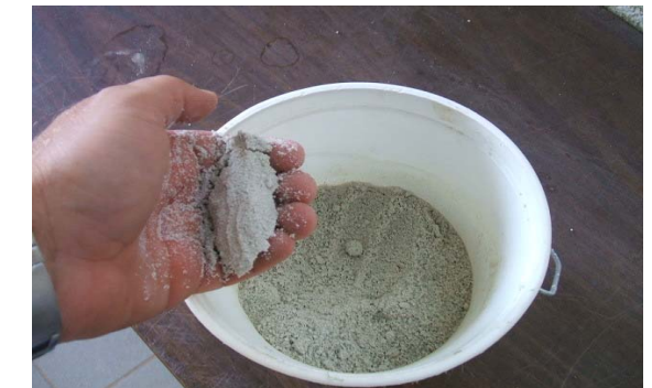
6. Mix hydrated with bonding agent
