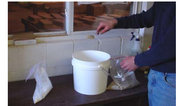
3. 5 parts aggregate, 1 part cement
